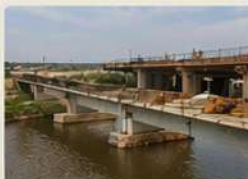
UNDER CONSTRUCTION PULL
